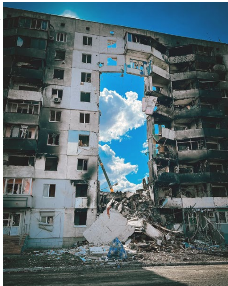
A destroyed residential building in Ukraine.
